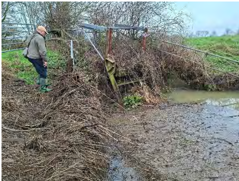
Photo 13. Top-hung tidal gate at the confluence with the Ouse. Functional or derelict? These gates will have a profound impact on the ecology of the lower section of the stream and the species that need to navigate in and out of the system.
