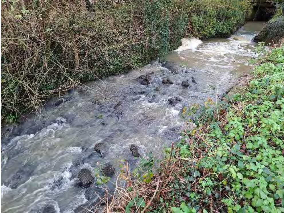
Photo 2. A typical bridge culvert on the Northend stream. These can be difficult for fish migration, but this example looks to have received a pre-barrage of imported rocks, designed to help drown out the invert of the culvert and give migrating fish a better chance of making upstream progress.
