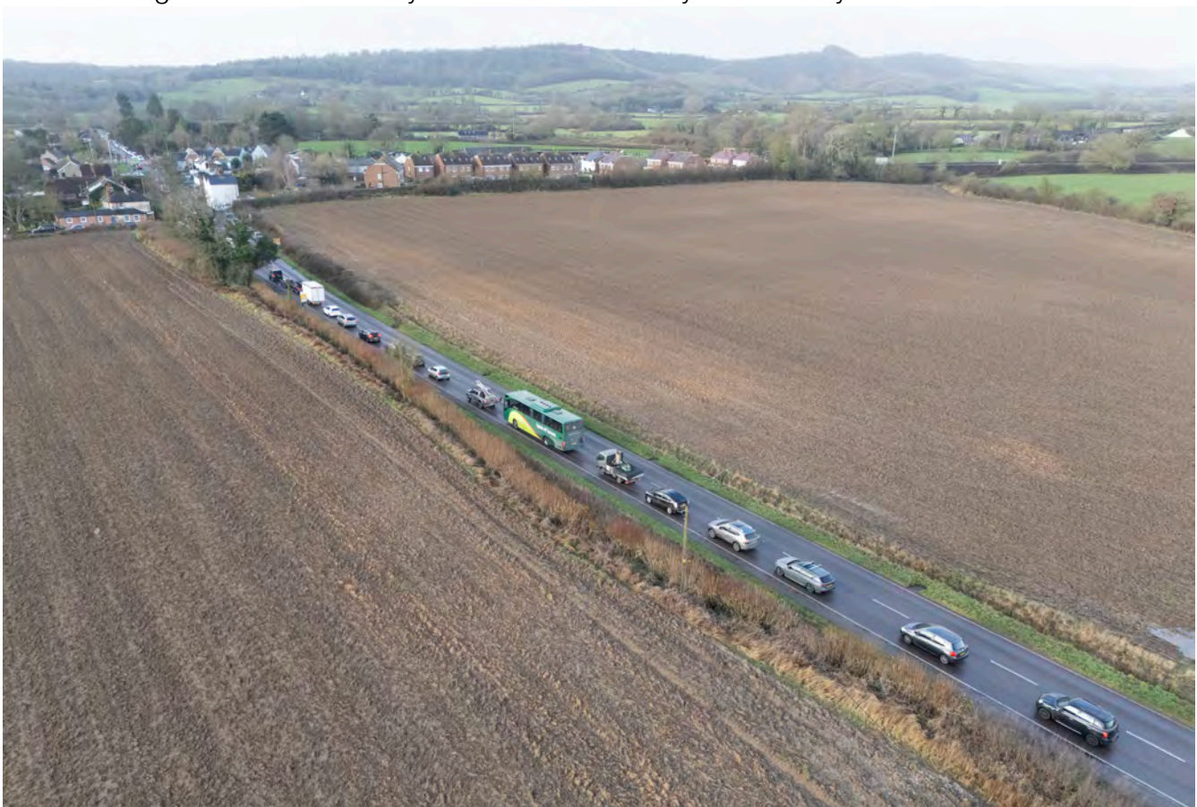
Photo looking South towards Level Crossing above East Field CB1. Thursday 12 th February 2026. 08:25
